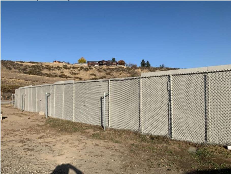
After the brush cutters did their part and the painters applied 25 gallons of paint, we have a nice start on our project.
